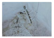
3. The sealant used to seal the parapet metal trims are cracking/deteriorating. These condition will allow water to enter the building at these areas. Recommendation-Install cap metal at missing cap section only. Clean and remove old sealant as necessary. Refasten laps if necessary. Seal all laps with high grade polyurethane roof sealant.
