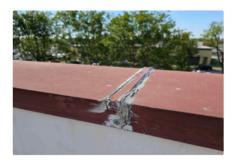
**4.** There is debris on the roof surface that is blocking proper water flow throughout the roofing system. Recommendation- Clear all roof debris and dispose of off site.
